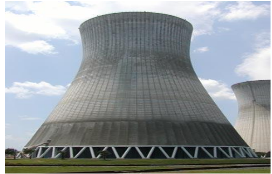
Fig-3 -Natural draft cooling tower [4]
