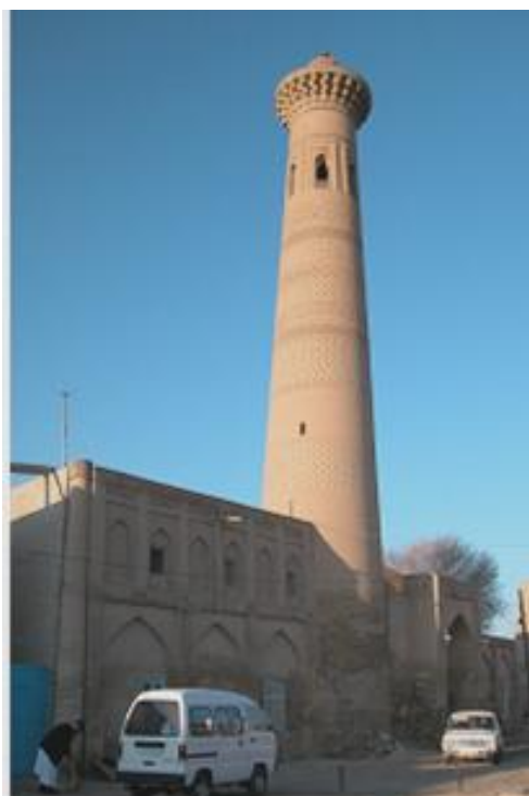
Figure 2. Minaret was damaged due to Minaret the man-made effects
