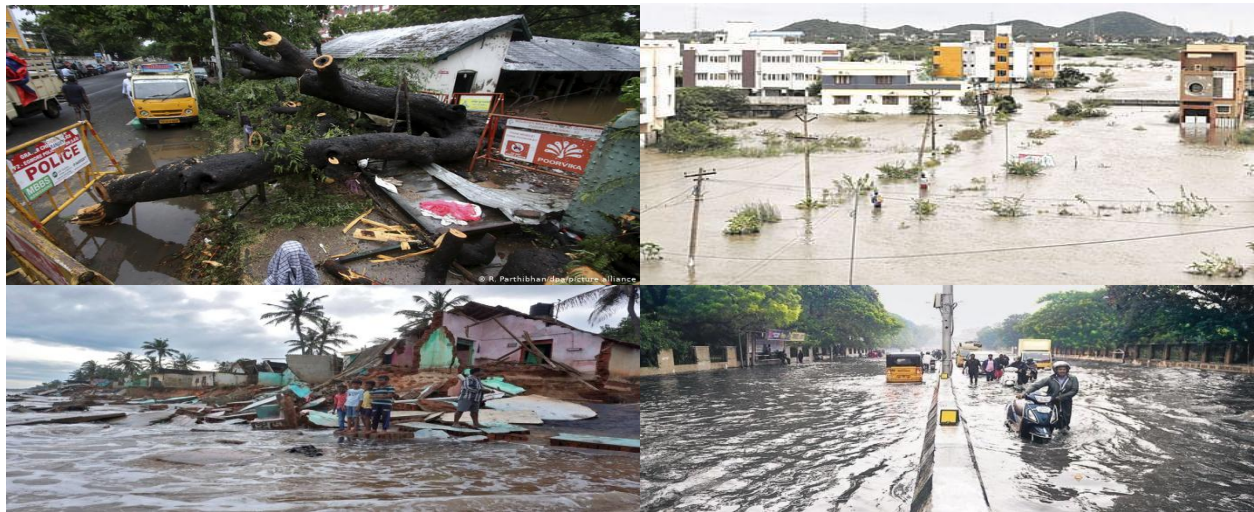
Image 8: Nivar cyclone damages
